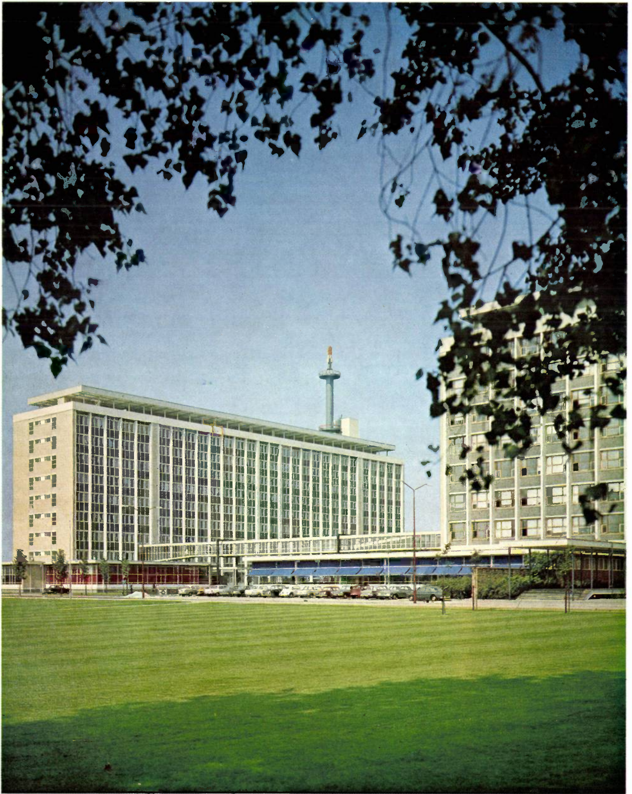
This "universal" laboratory building (WY) on the Waalre complex of Philips Research Laboratories has been in use since 1968. On its roof, on the right-hand side, there is an aerial for the experimental colour-television station. The following article gives an account of the buildings and also of the planning and development of the laboratory complex.
