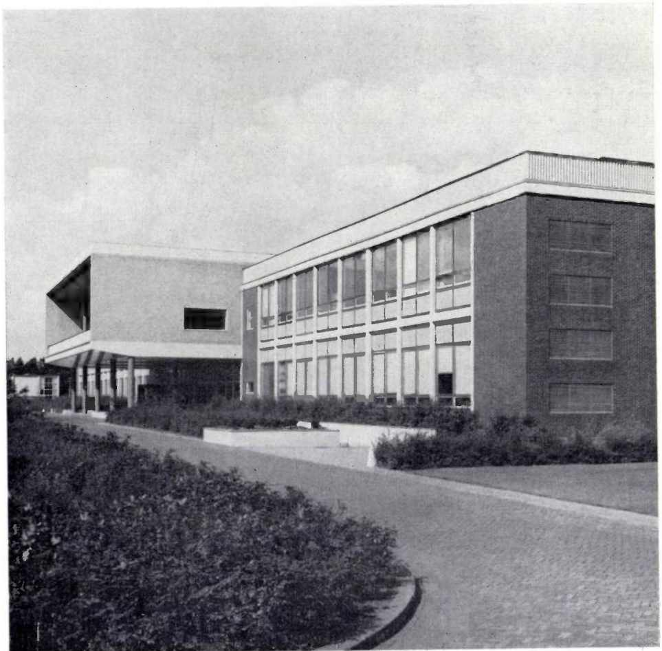
Building WA. Above: a plan of the ground floor; the three garden courtyards and the service roads to the basement are shown shaded. Right: the west front of the building, with the cafeteria projecting over the main entrance. The photographs opposite show the hall and one of the garden courtyards.
