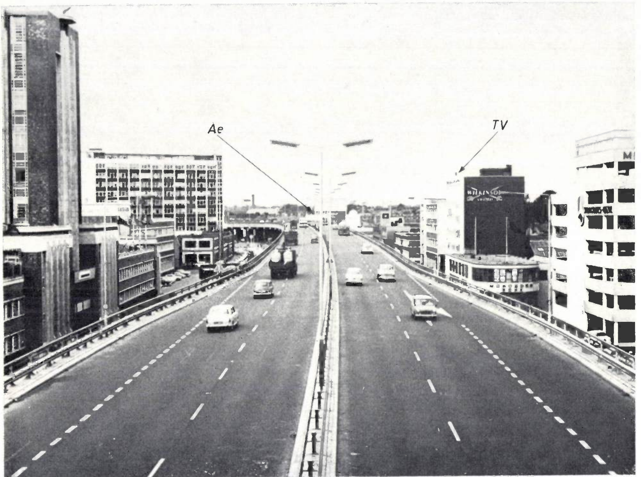
Fig. 6. The radar surveys the three left-hand lanes from the gantry to the slip-road (lower left). The positions of the radar and the television camera are marked Ae and TV .
